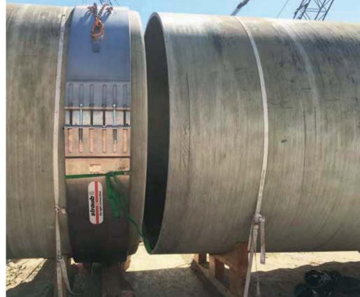
Strip inserts are used in case of: large distance between pipe ends, swelling due to agressive liquids, vacuum, under outside pressure, high temperature. Strip inserts are extras and must be ordered seperately.
