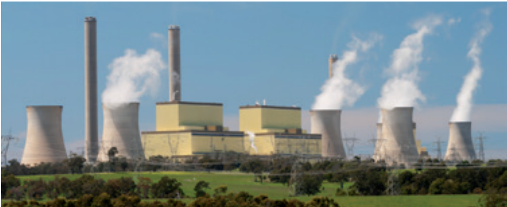
Coal Fired Power Station
