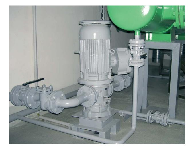
Vertical Selfpriming Side-Channel Pumps
