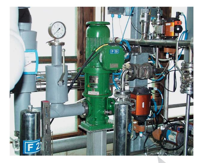
Sealless Magnetic Coupled Vertical Self-Priming Side-Channel Pumps
