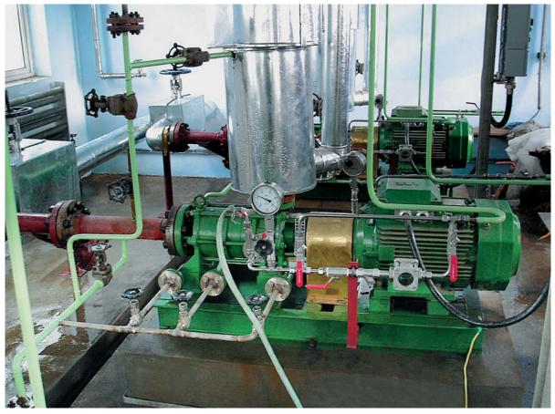
Heavy Duty Self-Priming Side-Channel Pumps Type SC
