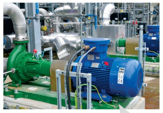
Sealless Magnetic Coupled Centrifugal Pumps acc. to EN 22858 / ISO 2858 Type NMR
