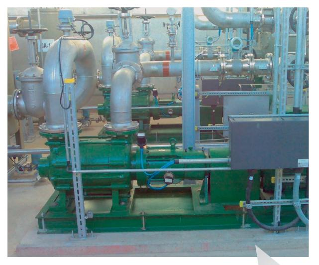
Sealless Magnetic Coupled Multistage Centrifugal Pumps with Priming Stage Type HZSM / HZSMB / HZSMR / HZSMA / HZSMAR our contribution for environmental protection
