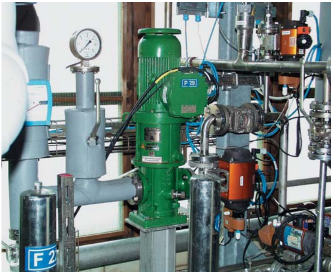
Type SMV with magnetic coupling. Liquid: Chemical Waste Water.
