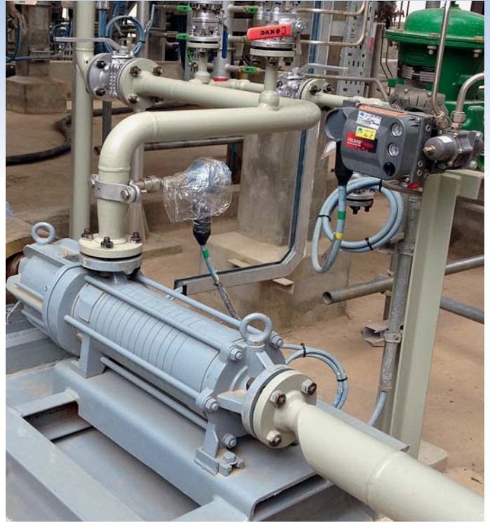
Type SCM with magnetic coupling. Liquid: Acrylonitrile, 45°C (113°F).
